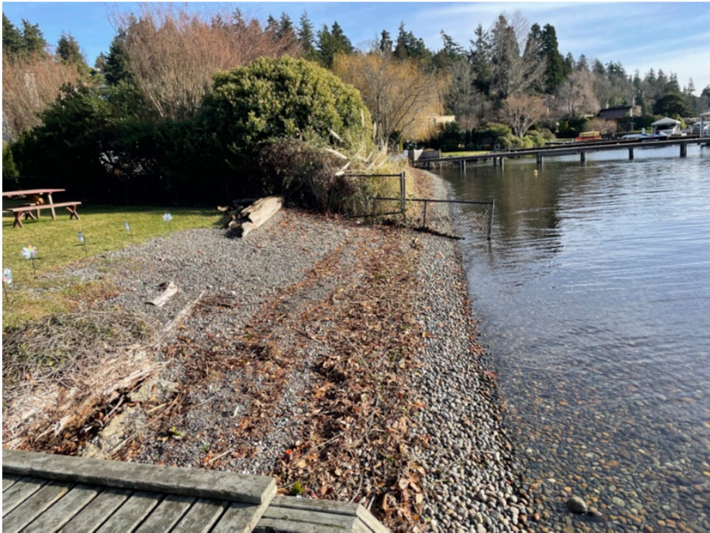
Photo 3 - Existing shoreline conditions looking south.
